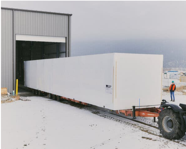
A completed module is towed from the facility.
