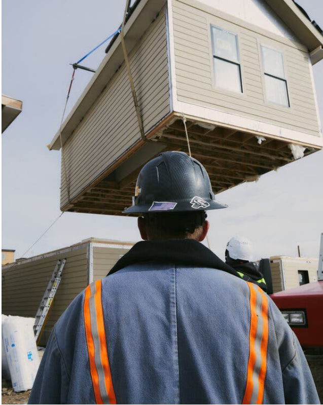
Cranes swing prefabricated housing units into place.
