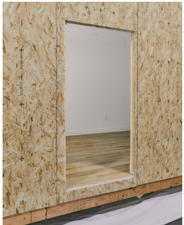
Finished houses consist of a few prefabricated boxes.
