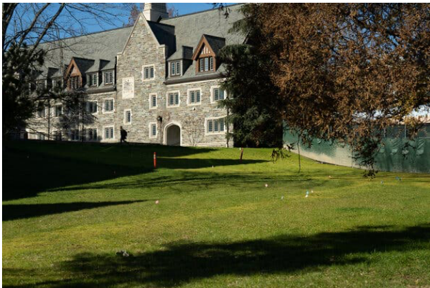
The tranquil surface of Prince University's campus sitting atop the new geoexchange system. Credit...Maansi Srivastava/The New York Times
