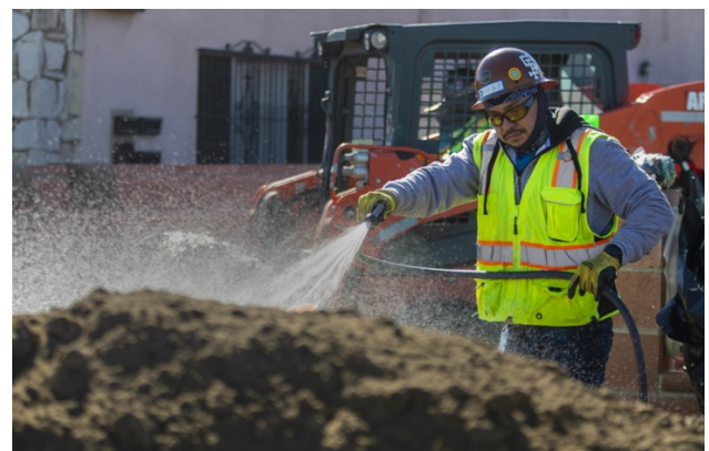
A worker sprays water on a pile of soil during lead remediation work in Maywood in November. (Francine Orr / Los Angeles Times)
